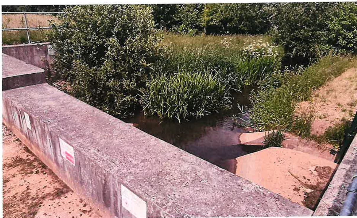
Figure 1-2. Outlet conditions on Vortex Flow Control Structure on a UK EA flood scheme (typical low flow conditions).
