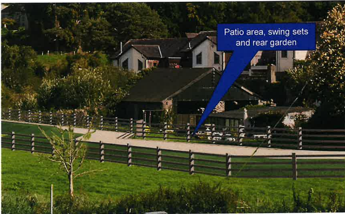
Figure 7-3: Blow-up of photomontage (in EIAR, Appendix 4.3) showing the defences to the rear of Walsh' property.
