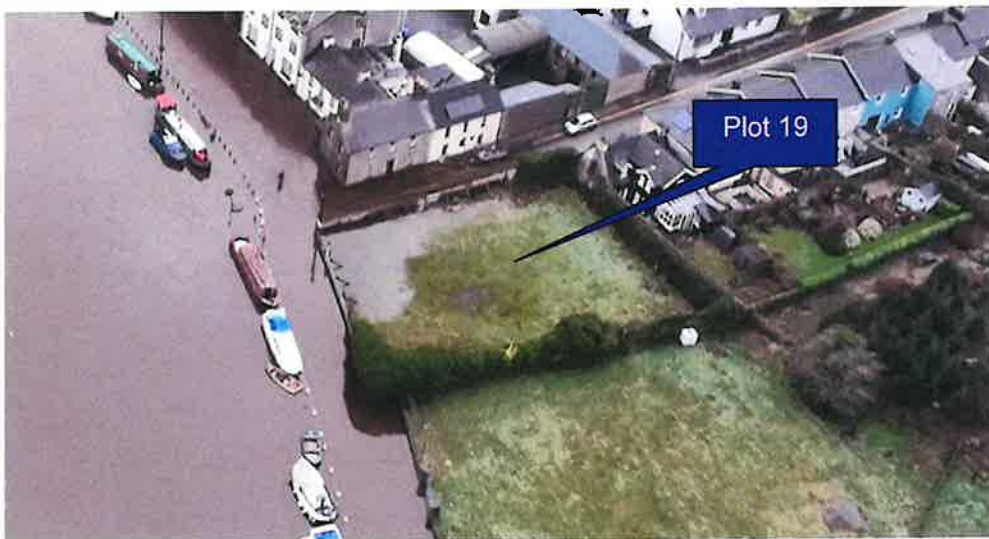
Figure 6-1: Flooding of Plot 19 in January 2019 – estimate to be a >10-year return period.
